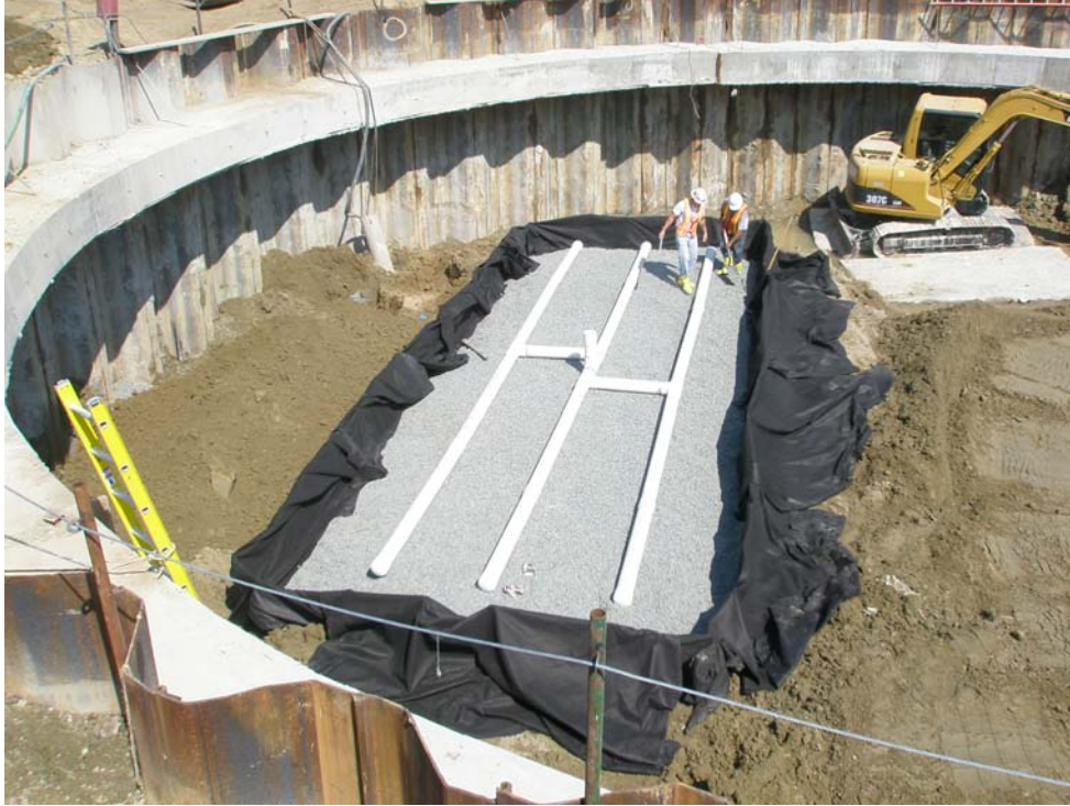
Photograph 3 – Installation of Infiltration Gallery in Western Portion of Excavation
