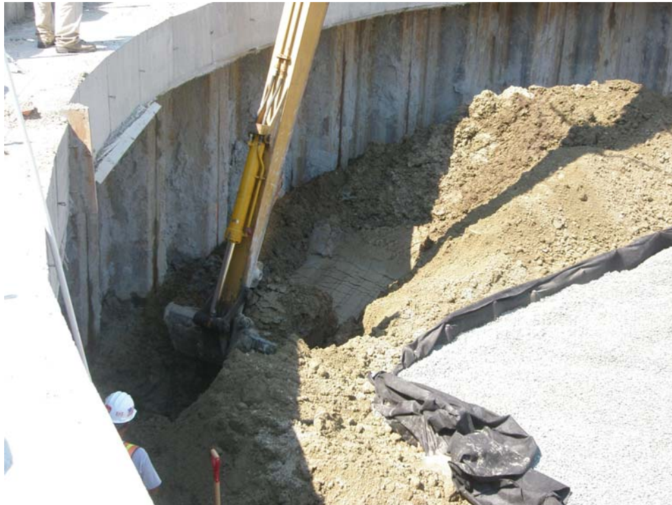
Photograph 2 – Final Area Excavated
