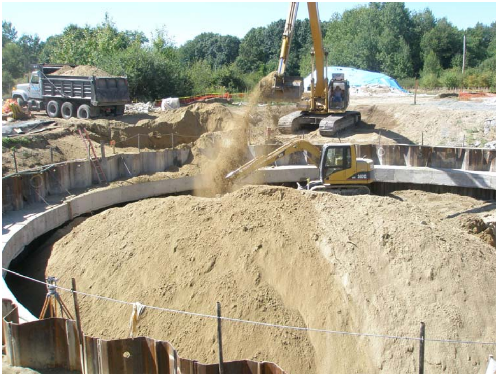
Photograph 4 – Backfilling Excavation
