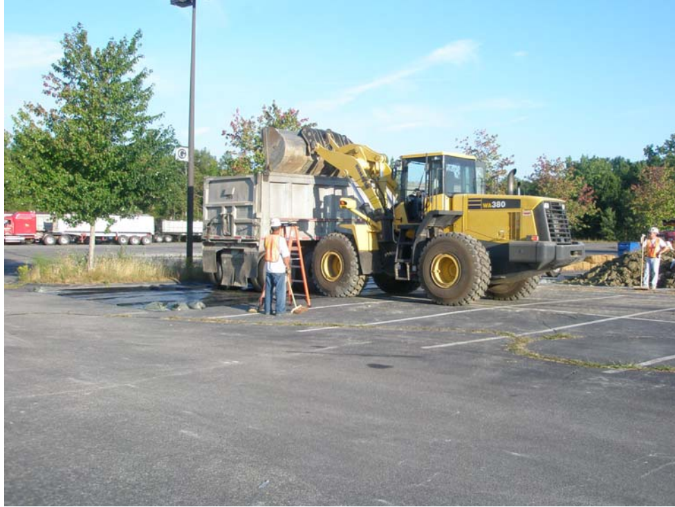
Photograph 1 – Loading Trucks for Off-Site Disposal
