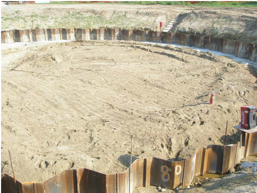
Photograph 6 – Backfilled to Approximately 119' ASL
