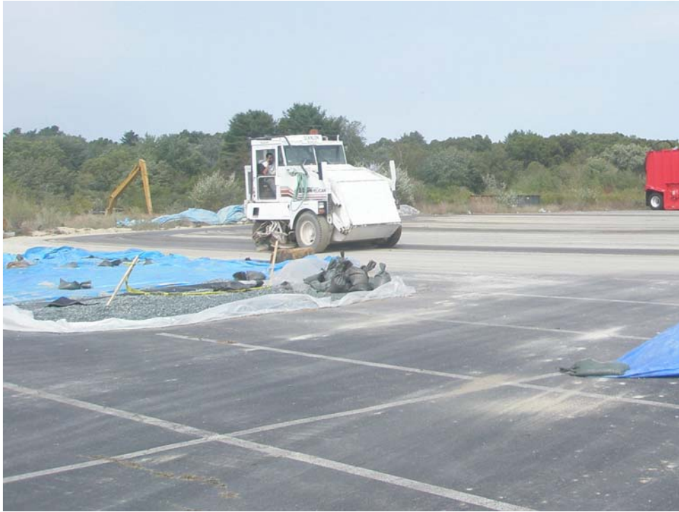
Photograph 5 – Sweeping Parking Lot and Former Soil Staging Areas
